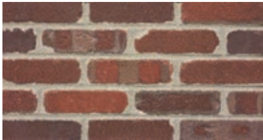
Standard 3/8" Mortar Joint
