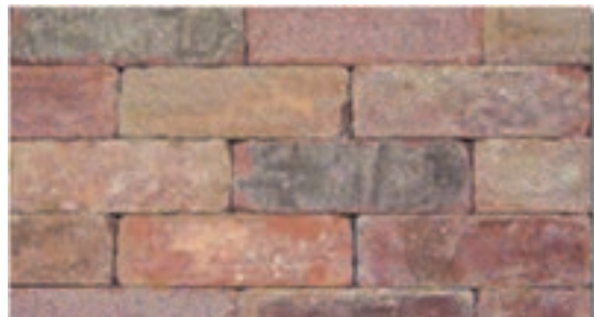
No Mortar Joint (Dry-Stacked)
