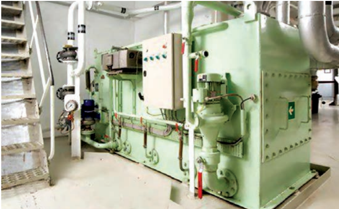
sewage treatment plant
