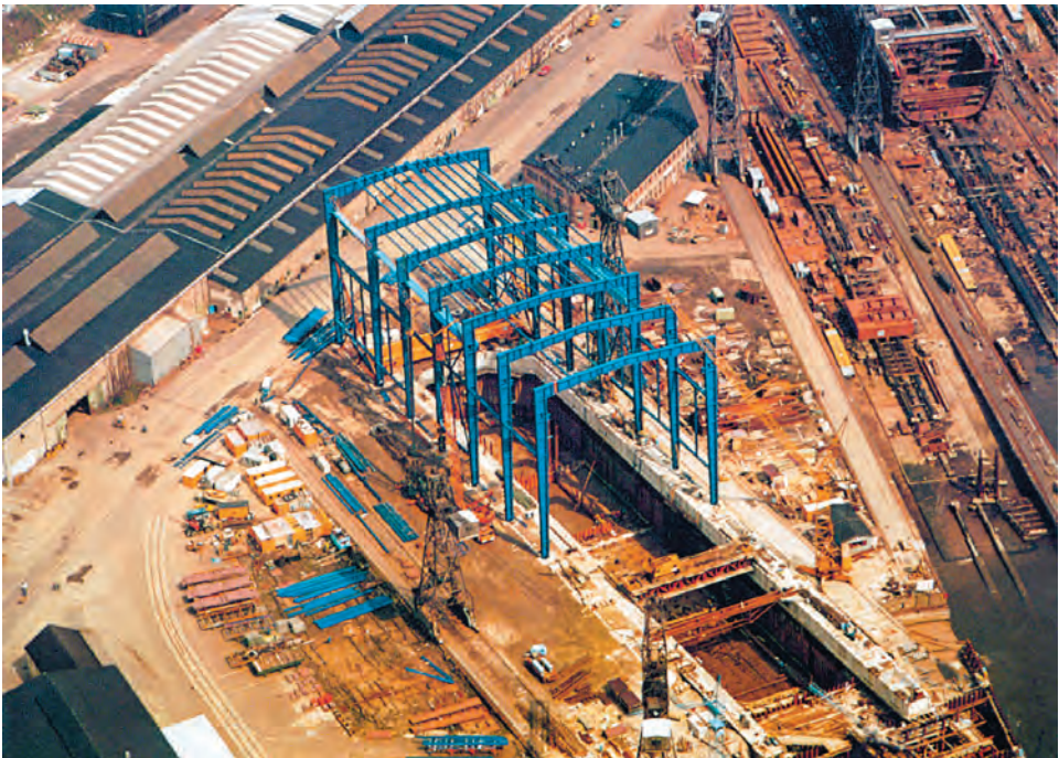
Covered graving Dock "D" during construction
