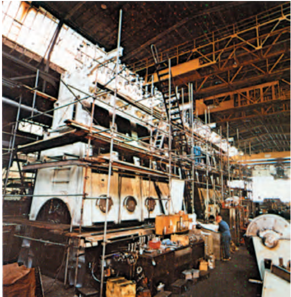
Assembly of a main Diesel motor
